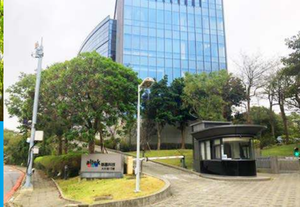
Altek main entrance
