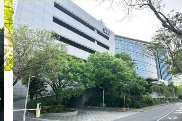
Aitek side entrance
